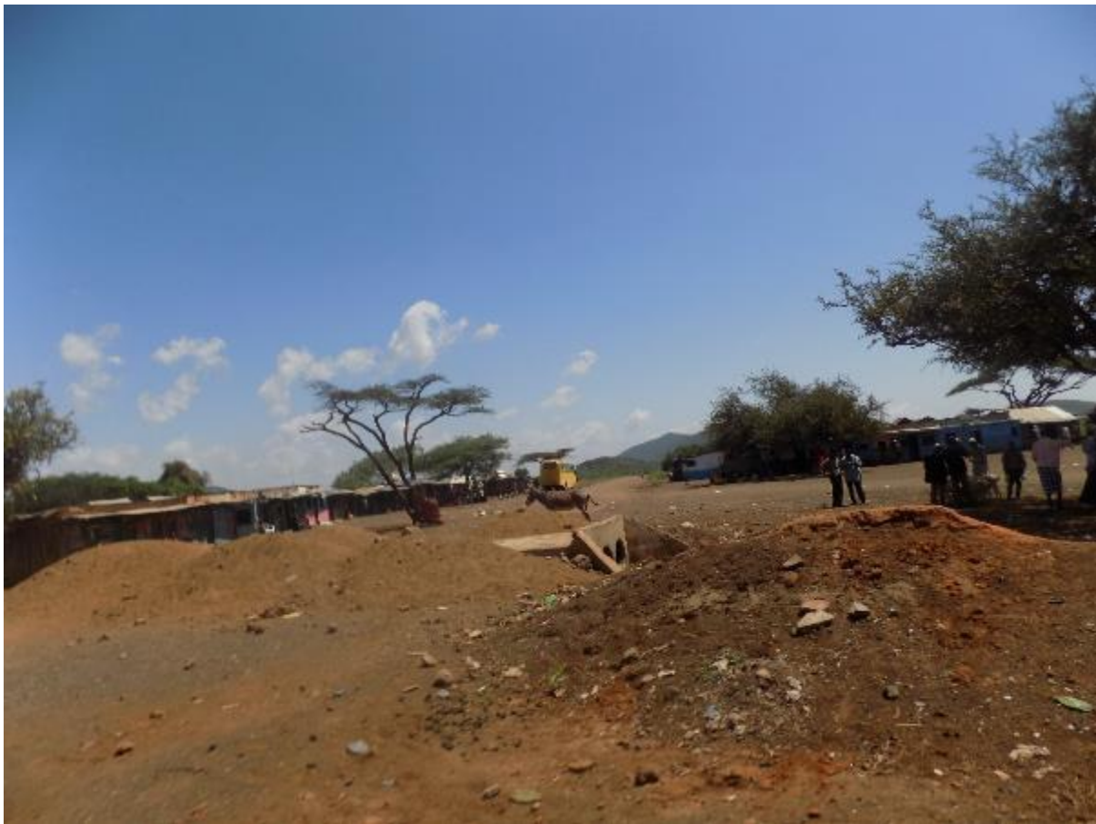
Figure 4-16: Typical Settlement (Kachuru) along the Project Road
