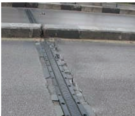
Cracks on post cast concrete
