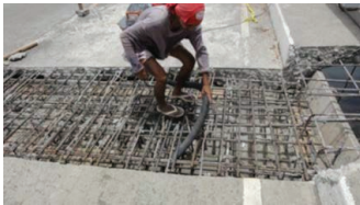
Placement of additional rebar and cleaning
