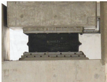
Rubber bearing (damaged)
