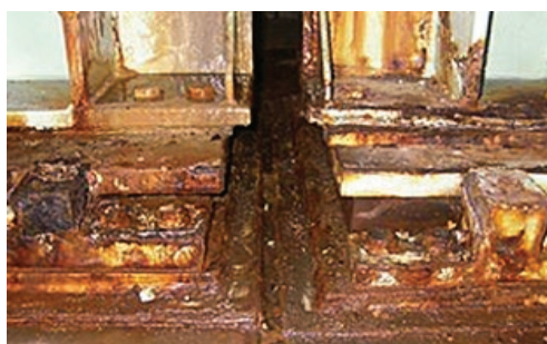
Girder ends with frequent water leakage
