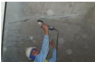
Cleaning Cracks
