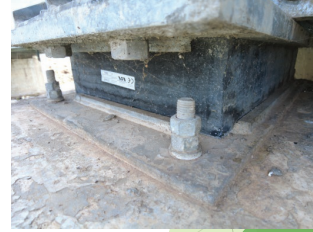
Elastomeric bearing used on Mbita Bridge
