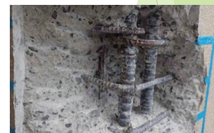
Corrosion condition
