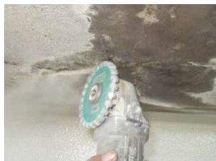
Preparing grooves for Caulking
