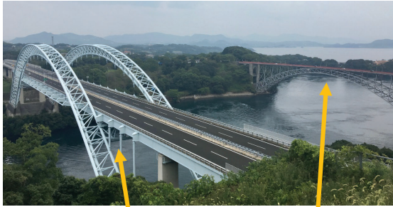
Left: Half-through bridge Right: Deck bridge
