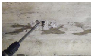
Removing loose particles
