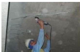
Curing of Injected Material
