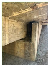
Siltation/Sedimentation on the bridge seat
