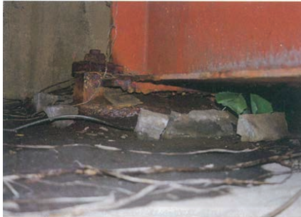
➤ Broken mortar seat
