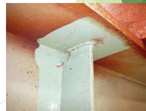
Cracks on steel member
