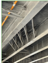
Deformation of steel girder/bracing
