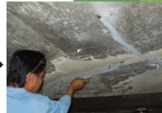
Drilling of holes and fixing injection pipes
