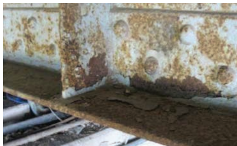
Corrosion of bottom flange
