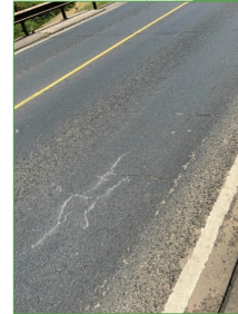
Crack on pavement
