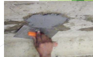
Placing Mortar
