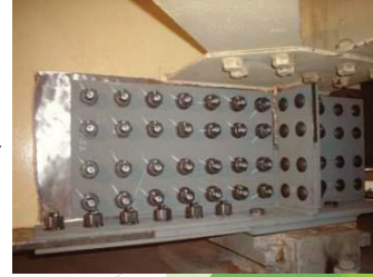
Steel plate added to the section
