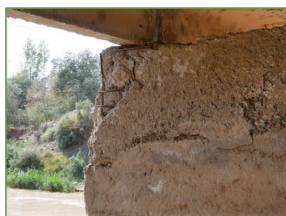
Sectional loss and Rebar exposure of pier concrete
