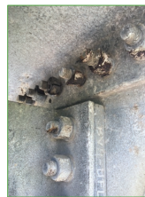
Missing and Corrosion of Bolts
