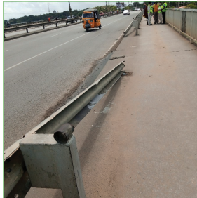
Damages on railings, guardrails, fences, and kerbs
