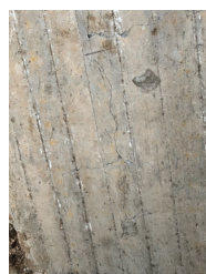
Cracks on the deck slab
