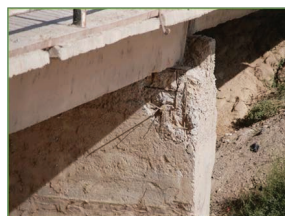
Sectional loss and Rebar exposure of pier concrete
