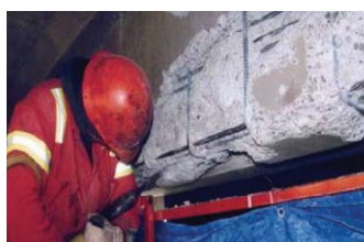
Removal of girder concrete
