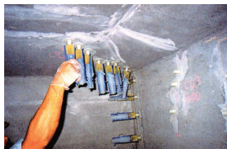
Epoxy injection work
