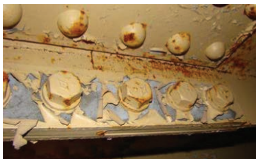
Deterioration of corrosion protection
