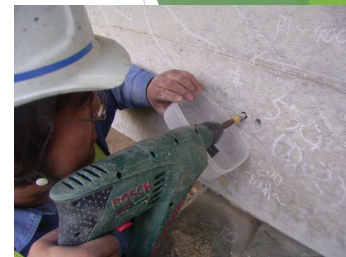
Drilling concrete
