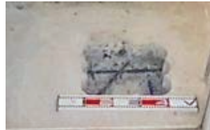
Rebar arrangement
