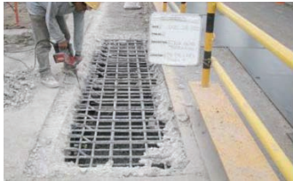
Removal of deteriorated deck slab
