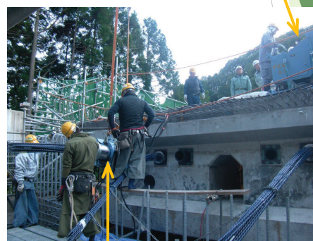
Tensioning work after the concrete hardens
