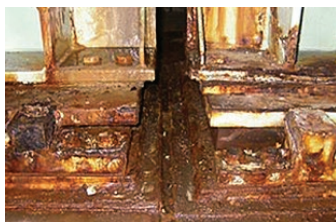
Corrosion of bearings
