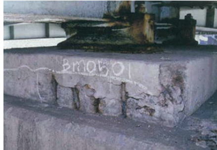
➤ Exposed rebars in the concrete bearing seat
