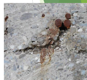
Cavity under the rebar
