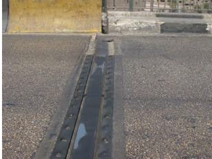
Rubber faceplate type: - Worn-out/damaged surface rubber
