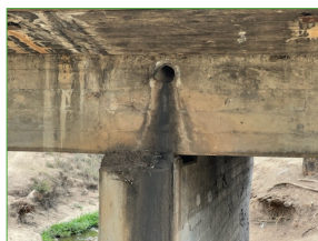
Siltation/Sedimentation on the bridge seat
