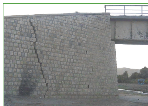
Cracks on the abutment/Retaining wall
