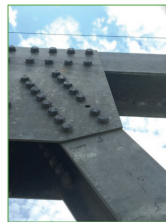
Missing and Corrosion of Bolts
