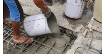
Pouring mortar from lower part to upper part
