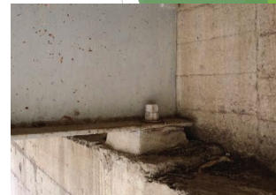
Bearings at the abutment fixed by anchor bolt.
