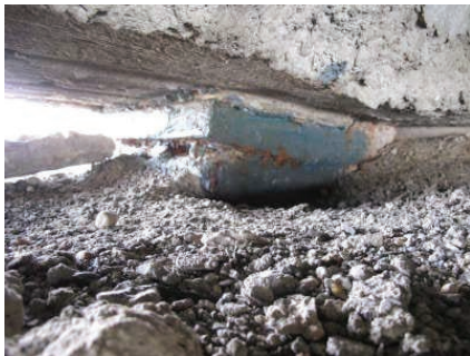
➤ Clogging/soil choking ➤ Reoccurrence of corrosion
