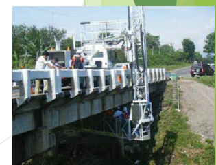
Cleaning using water pressure
