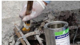
Applying epoxy bonding material
