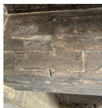
Rebar fractures and cracks on the main girder/cross beam
