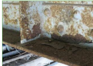
Corrosion of steel girder
