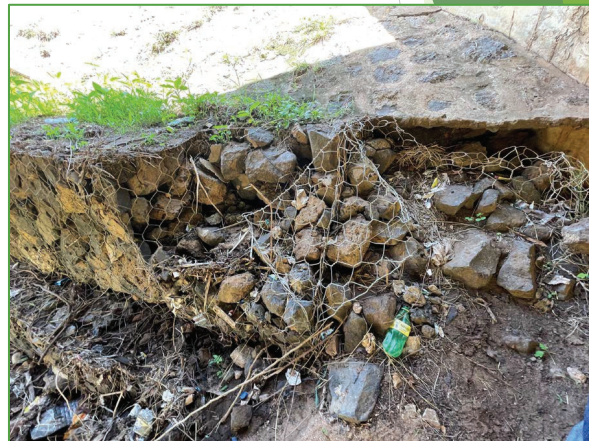
Dilapidated gabion mesh
