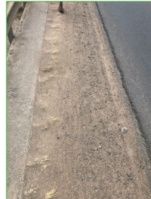
Clogging of the drainage facilities
