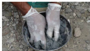
Mixing right proportions of cement powder and emulsion
