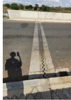
Expansion joint on Tiva Bridge Reliever
