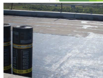
Construction of waterproof layer using membrane sheet on concrete deck slab.
