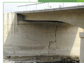
Cracks on the abutment/Retaining wall
