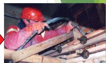
Grouting Mortar after setting formwork
