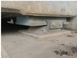
Sliding steel bearing used on Kilifi Bridge
