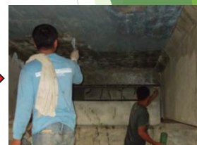
Applying mortar using trowel or brush
