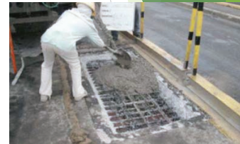
Casting new concrete
