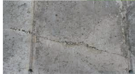
Cold Joint on abutment
