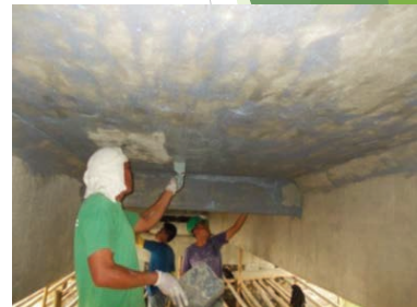
Application of protective coating
