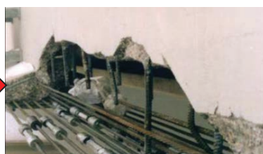
Cutting of deteriorated rebars and adding new rebars
