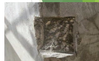
Preparation of repair section
