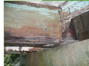
Corrosion of steel girder
