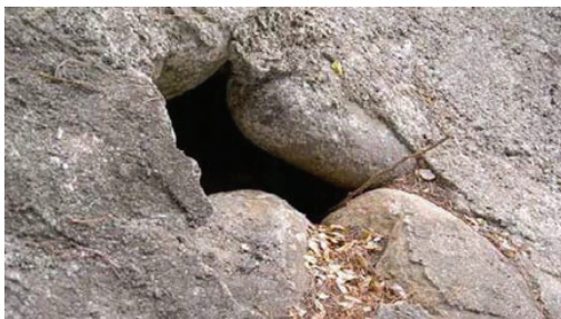
Missing stone on a masonry protection wall
