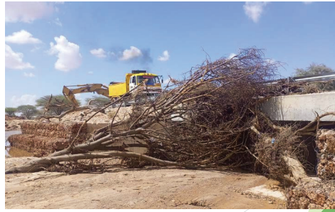
Accumulated driftwood obstructing the free flow of water
