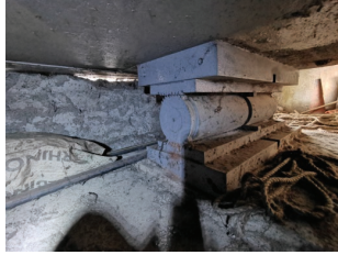
Roller steel bearing used on Nyali Bridge
