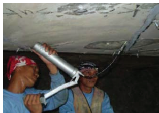
Injecting the Epoxy Grout
