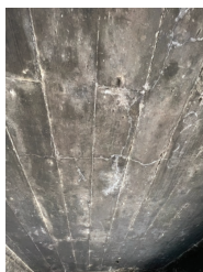
Cracks on the deck slab
