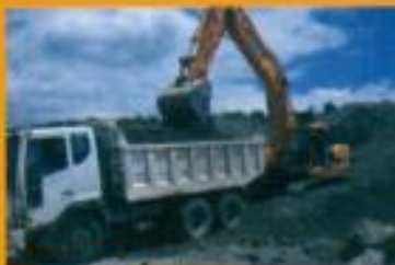
Dump Truck and Excavator
