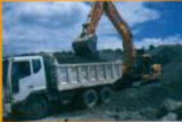
Dump Truck and Excavator
