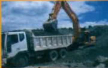
Dump Truck and Excavator
