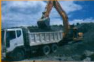
Dump Truck and Excavator
