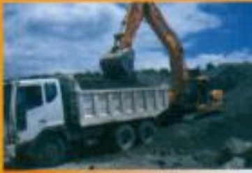
Dump Truck and Excavator
