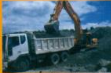
Dump Truck and Excavator
