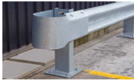
Buffer End Connection
