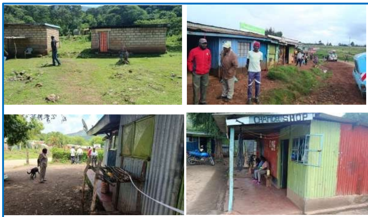
PhotoPlate 1:Some of the Structures That Will Be Impacted Along the Road Corridor
